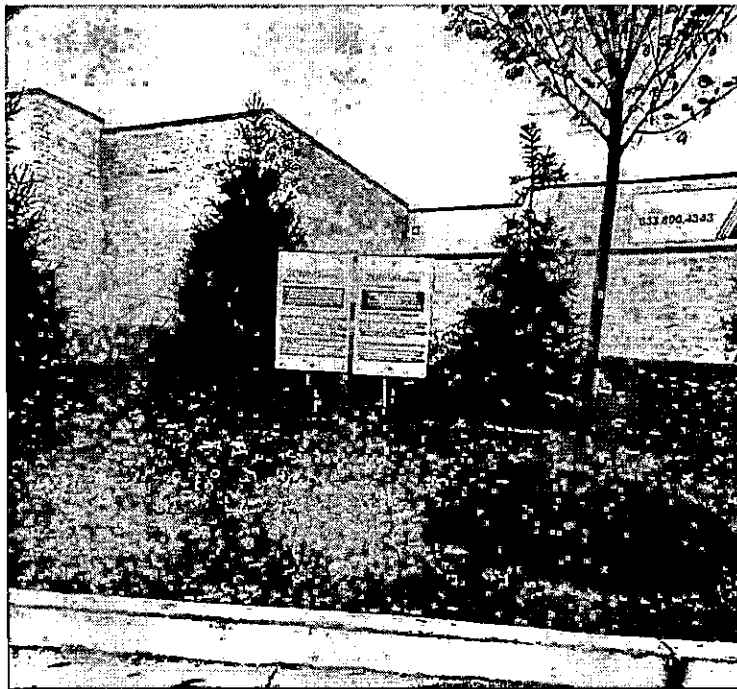
Second Set of Signs Back of Building 10240 (aka 10210) Mill Run Circle ~ 10/12/2020
