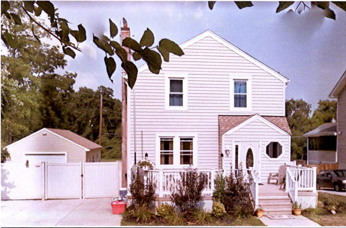
Front view of 5625 Ashbourne
