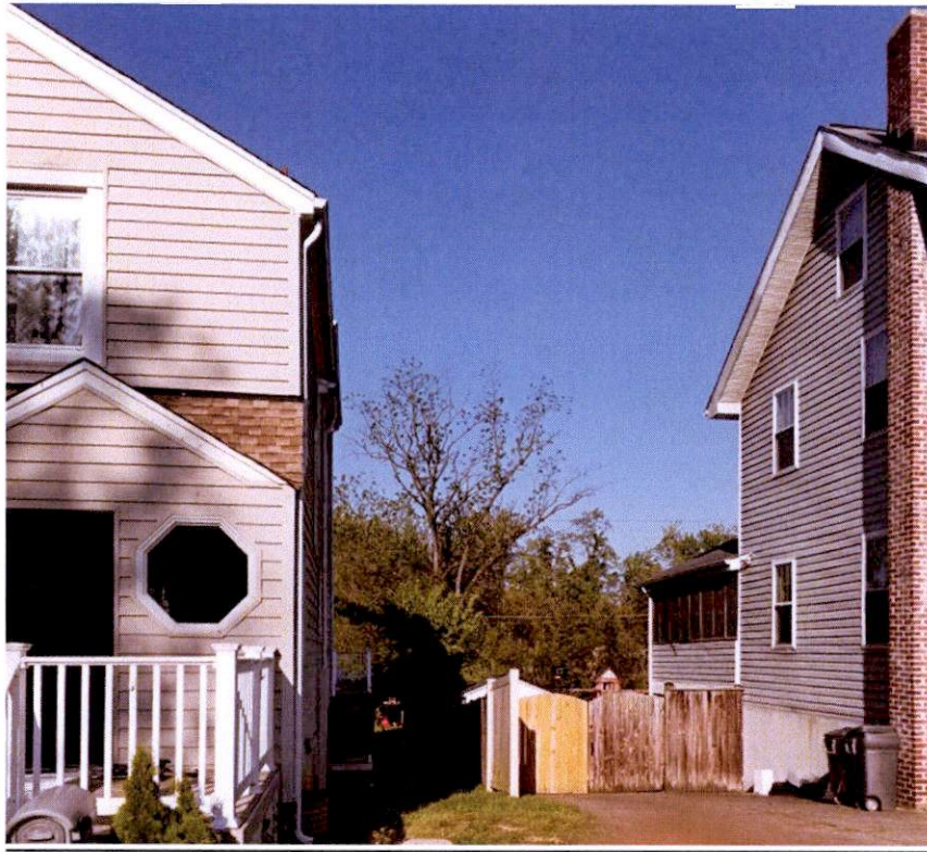
View of property line between 5625 & 5627 Ashbourne
