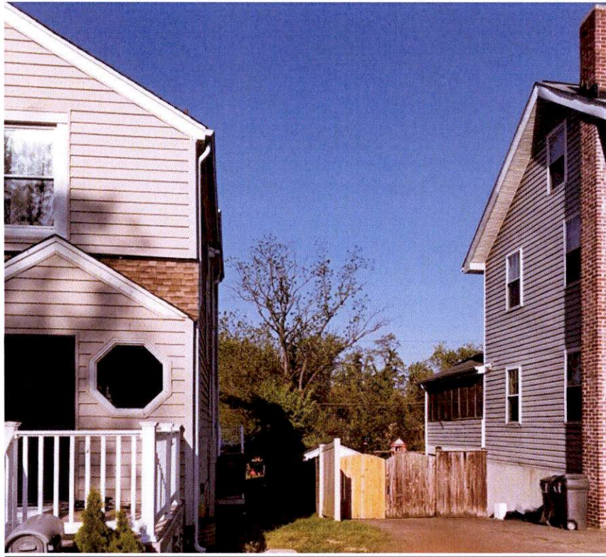
View of property line between 5625 & 5627 Ashbourne
