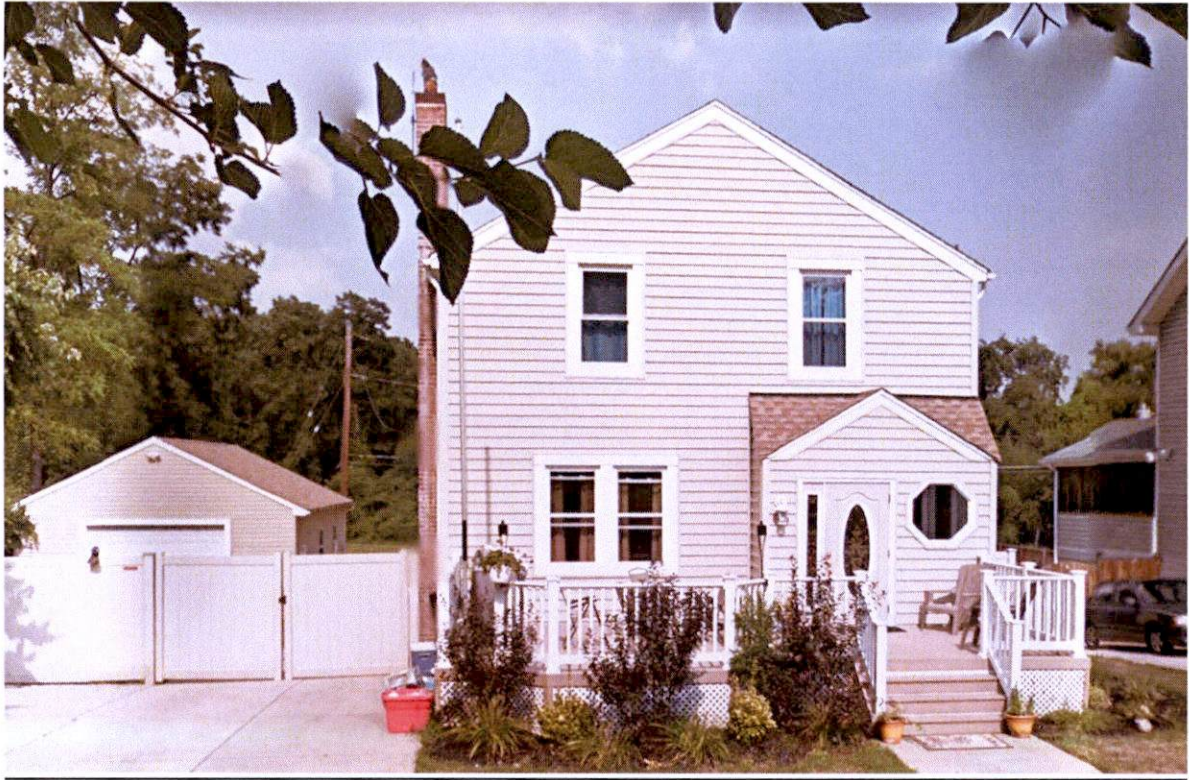
Front view of 5625 Ashbourne
