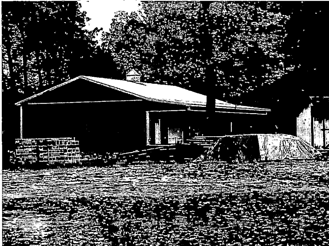
Garage on property behind this property at 1706 Hilltop Road, Case: 2013-0138-A
