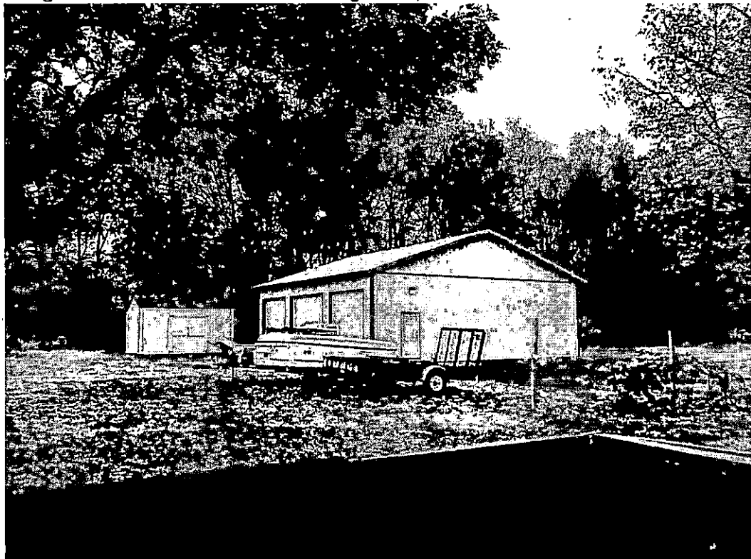
Garage south and east at 1703 Middleborough Road, Case: 2012-0280-SPHA
