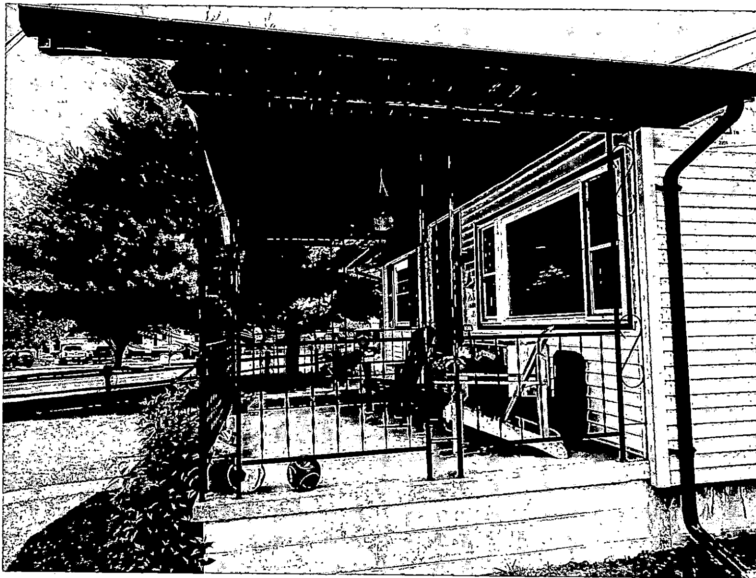
View across porch, looking southeast, toward Wilson Point Road.
