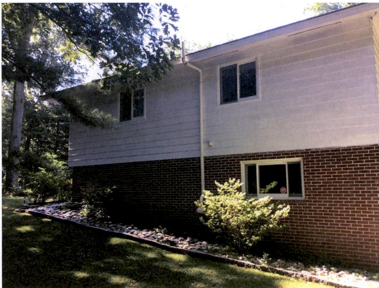
Photo 14: This photo is looking southwest towards the north side of the existing dwelling. Note slope of existing ground.
