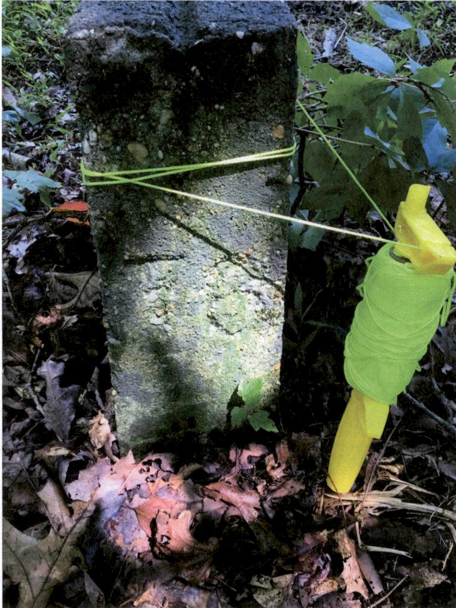
Photo 3: This photo shows concrete monument No. 76 as described in the property Deed and is the POB of the property line stake out.
