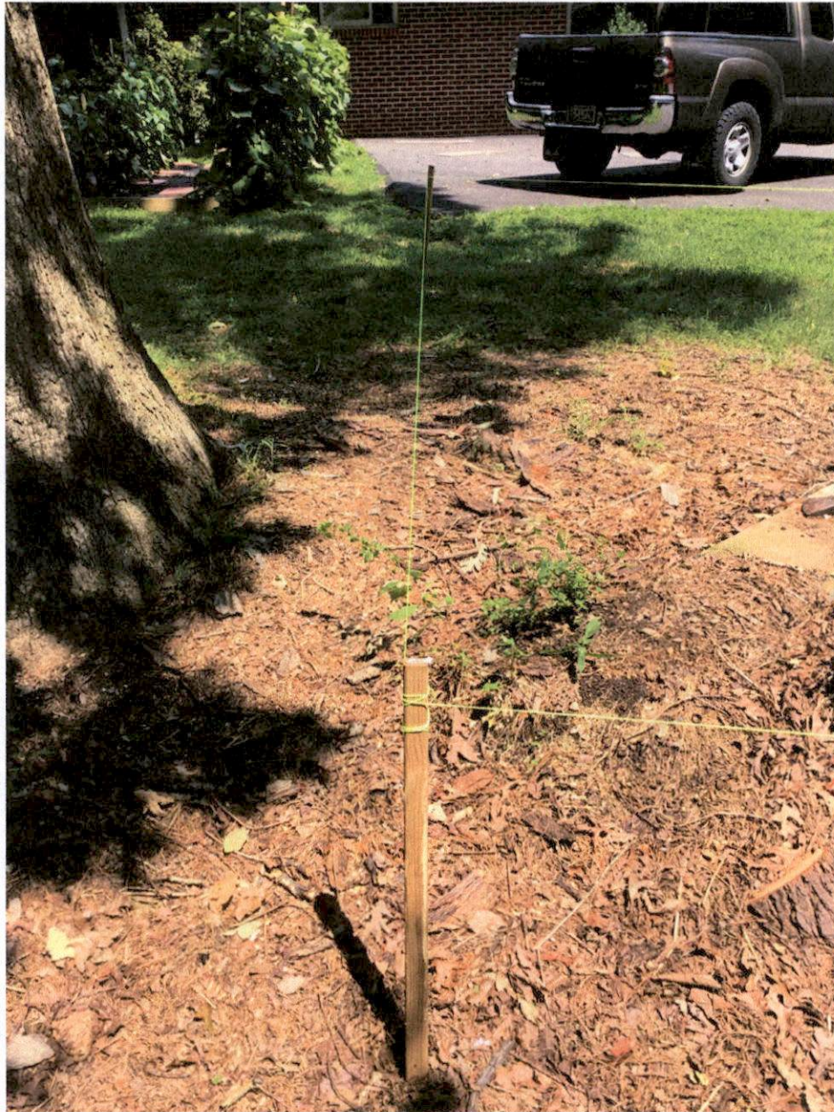
Photo 9: This photo is looking northeast toward the existing dwelling from the west corner of the proposed shed foundation. This photo shows the 2 foot offset from the existing 34" BHD white oak on the left. (The size of the shed has now been reduced to 12' X 18' and will have a 4 foot offset from the existing tree).
