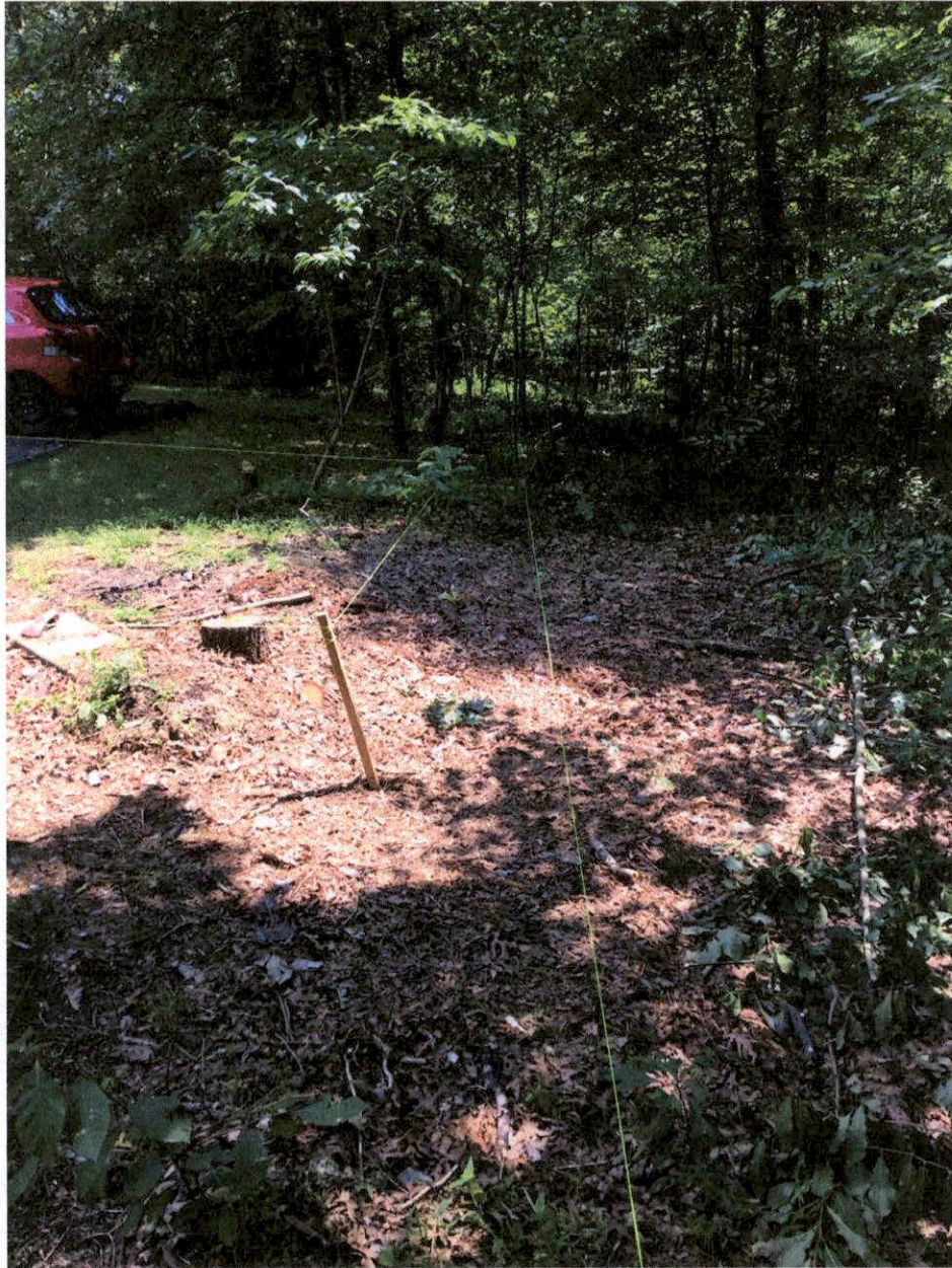
Photo 8: This photo is looking southeast toward the 2 nd POC adjacent to Spooks Hill Rd. from south east of the POB. This photo shows the stakeout of the proposed shed foundation and the 2 ft. setback.
