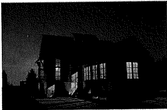
1466 BUTLER ROAD ACCESSORY BLDG
