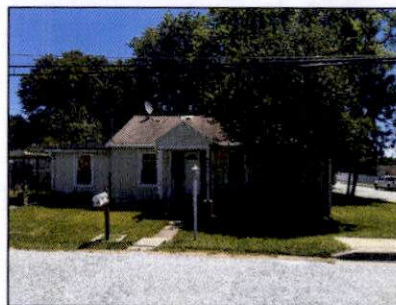
EXISTING FRONT VIEW
