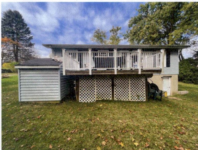
Photo #8: 125 Taunton Ave site of new proposed 16x22' deck with stairs (will be over rear door on right side)
