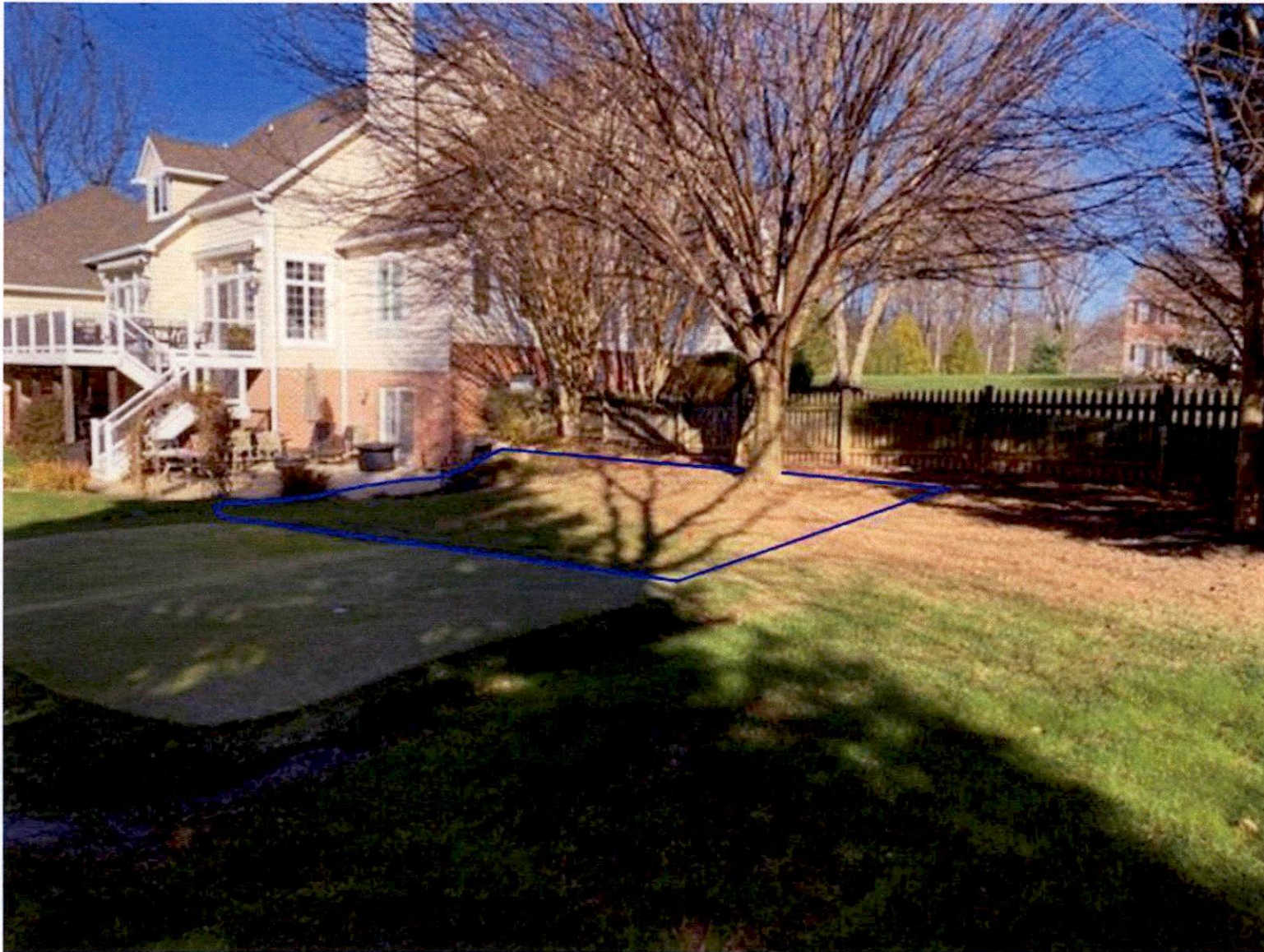
Photo 2 – From Southeast Property Corner, Looking Northwest towards Project
