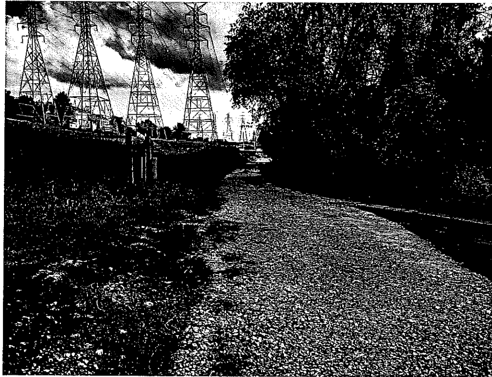
SHARED DRIVE WITHIN PRIVATE RIGHT-OF-WAY LOOKING SOUTHERLY TOWARDS MAGLEDT ROAD
