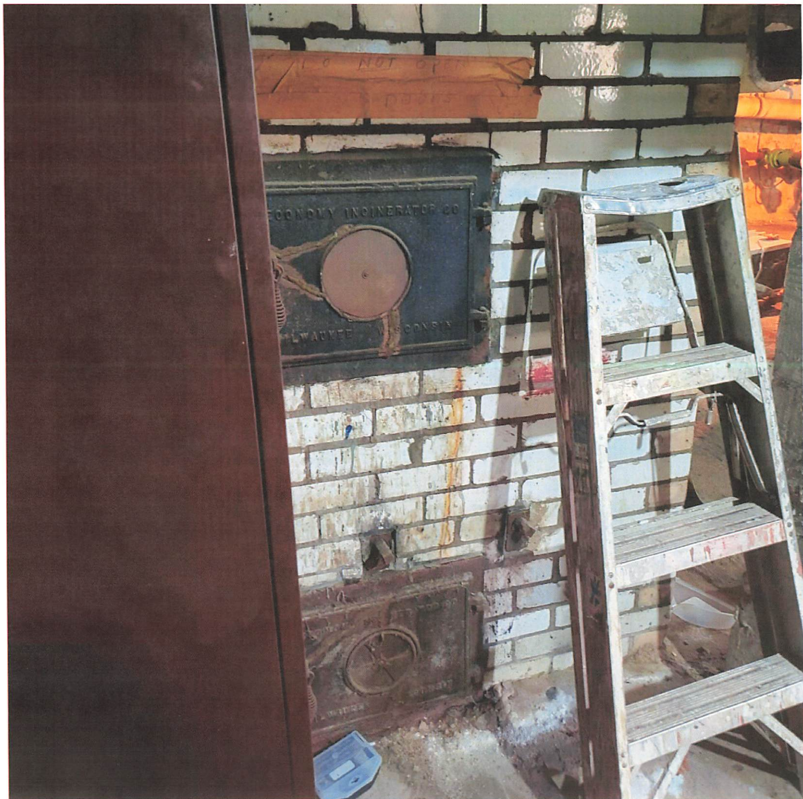
629 Plymouth Rd Base of old incinerator in the basement.
