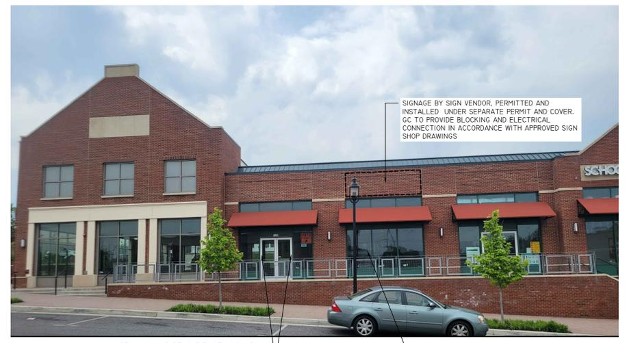
SIGNAGE BY SIGN VENDOR, PERMITTED AND INSTALLED UNDER SEPARATE PERMIT AND COVER. GC TO PROVIDE BLOCKING AND ELECTRICAL CONNECTION IN ACCORDANCE WITH APPROVED SIGN SHOP DRAWINGS.
