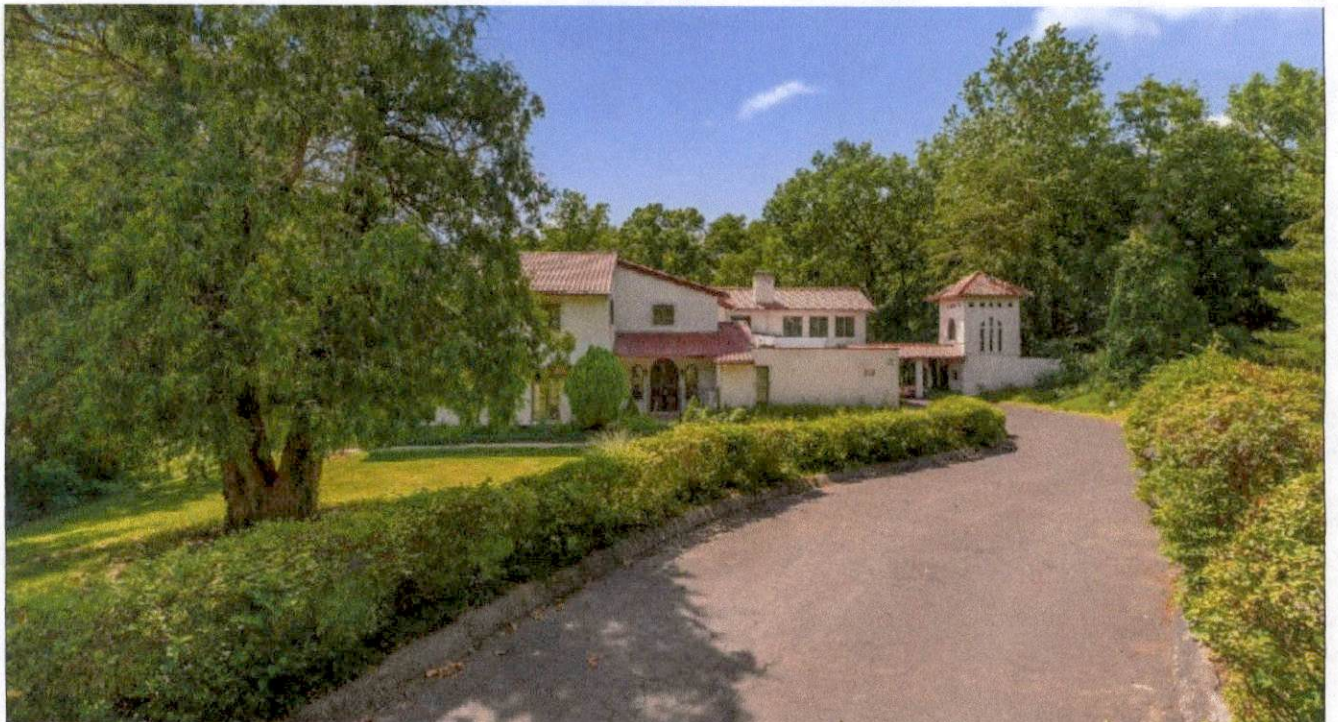
driveway view of 7 barranco
