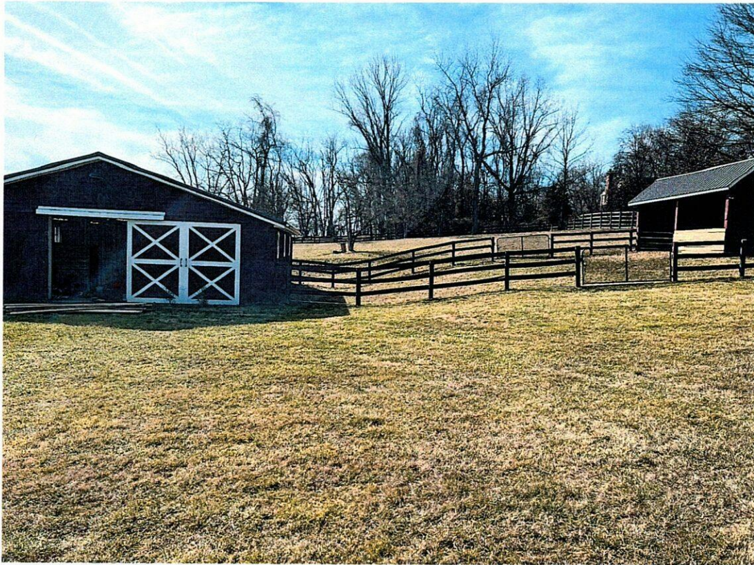
From garage facing west toward existing barn
