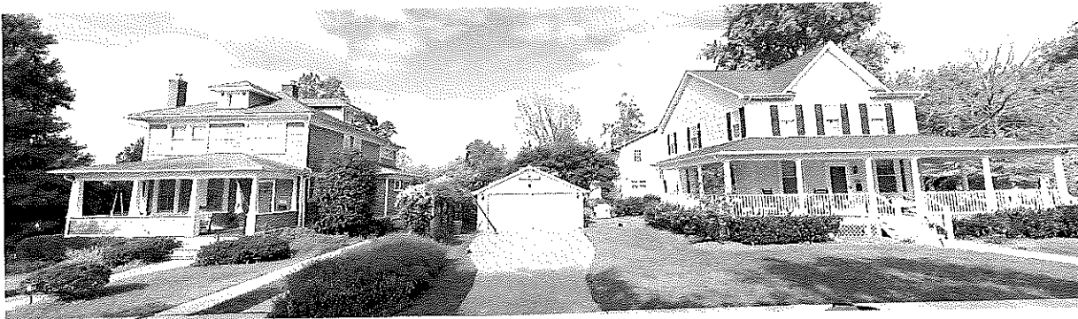
506 HIGHLAND AVE EX. GARAGE FRONT & PROXIMITY TO 504
