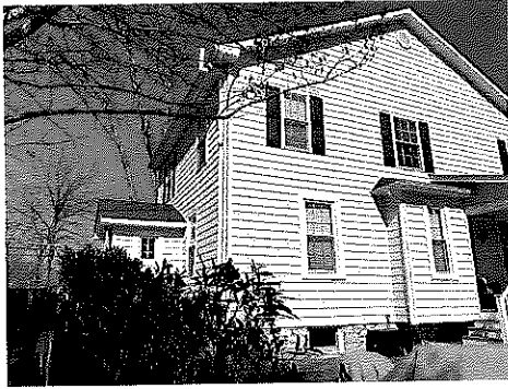
1 506 HIGHLAND AVE EX. LEFT REAR CORNER
