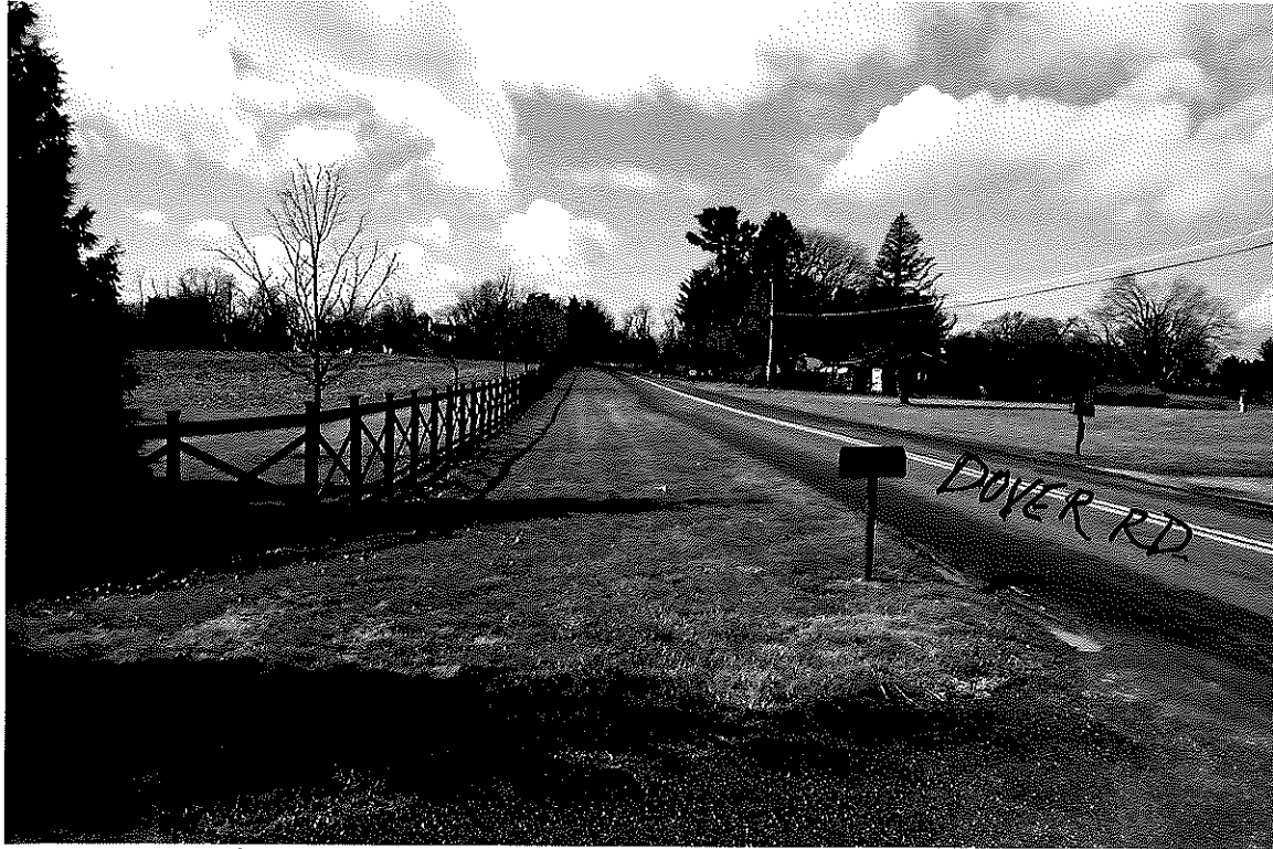
① DRIVEWAY LOOKING WEST
