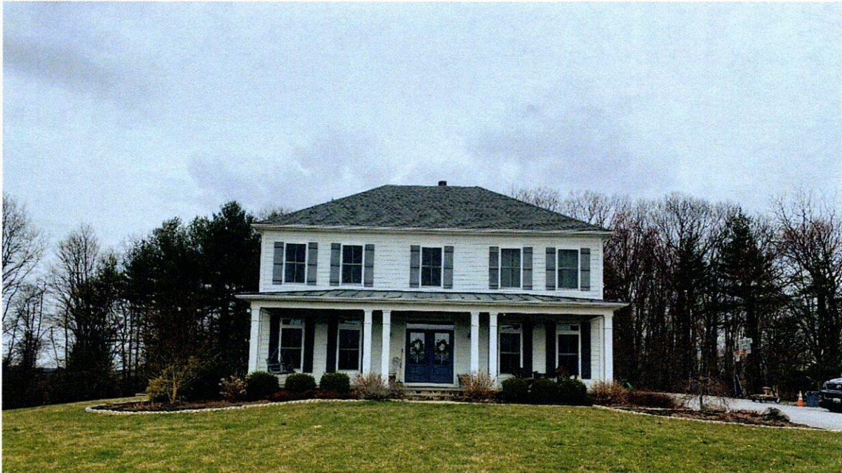
Front of Existing Structure:
