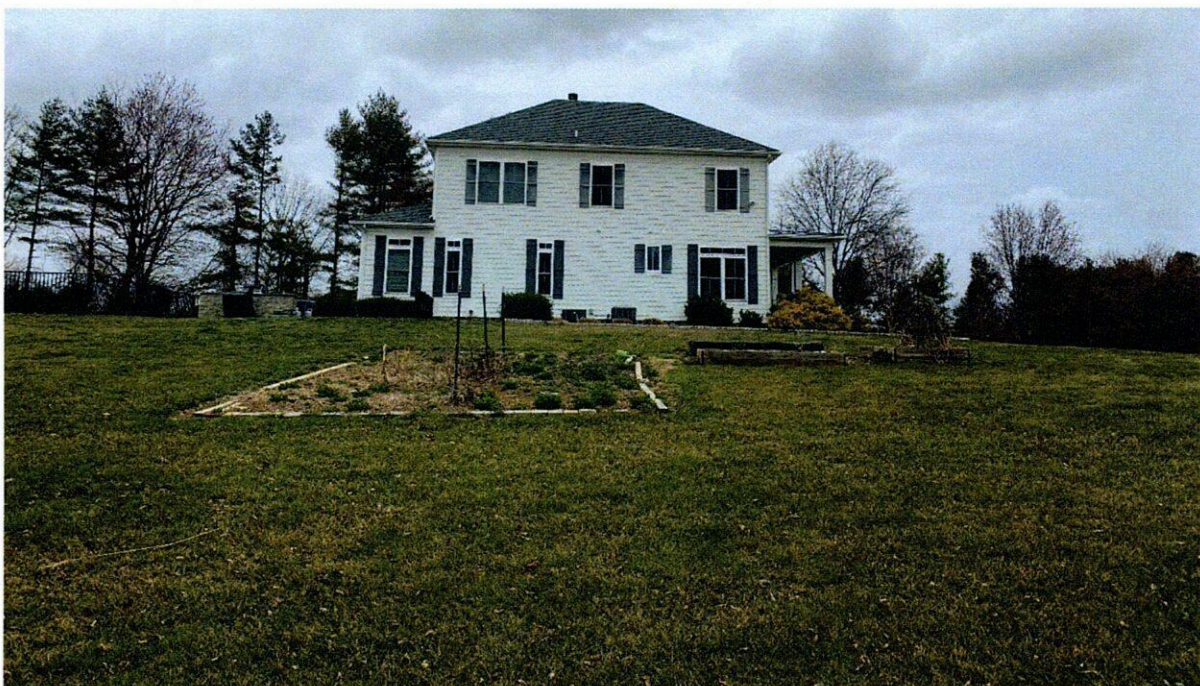
Left Side of Existing Structure (Showing Downhill Grade)
