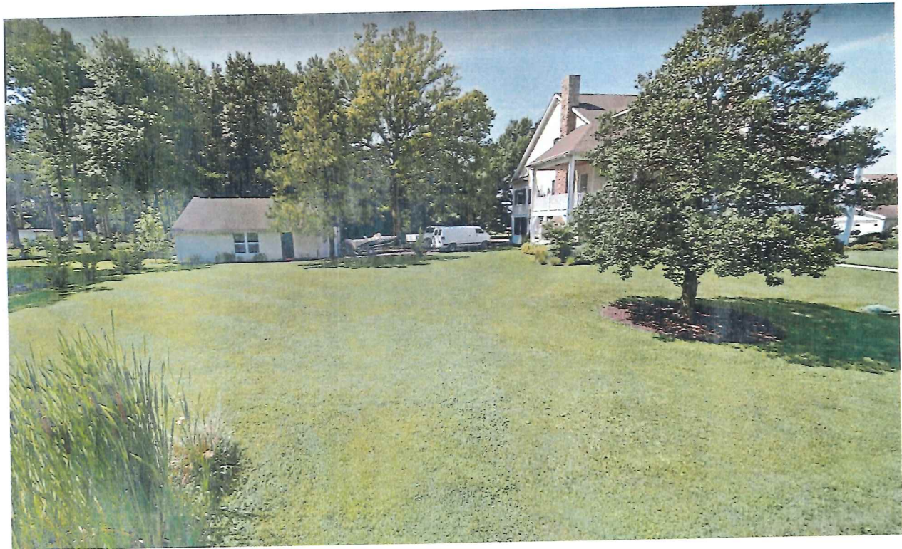
View from Burke Road to garage on left before it was damaged.
