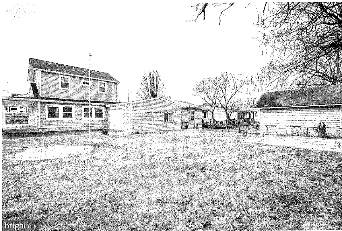
SIDE VIEW OF THE PROPERTY FROM RUNWAY CT
