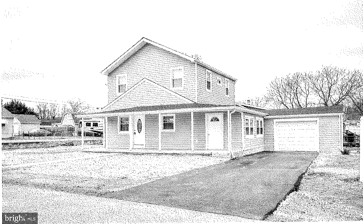
FRONT VIEW OF PROPERTY FACING RUNWAY CT
