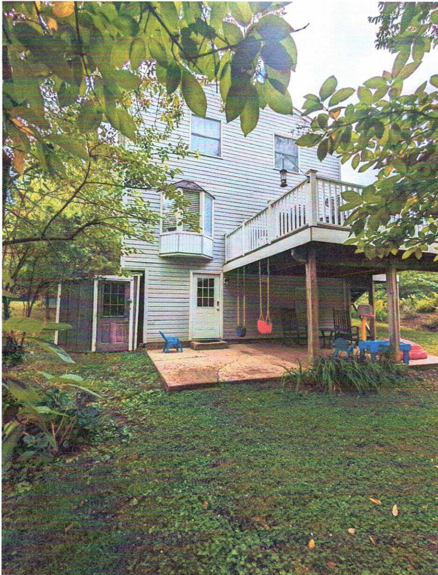
Above Photo: A final look at the back of 301 Locust Drive. The proposed screened-in porch would be extended the length of the concrete patio.
