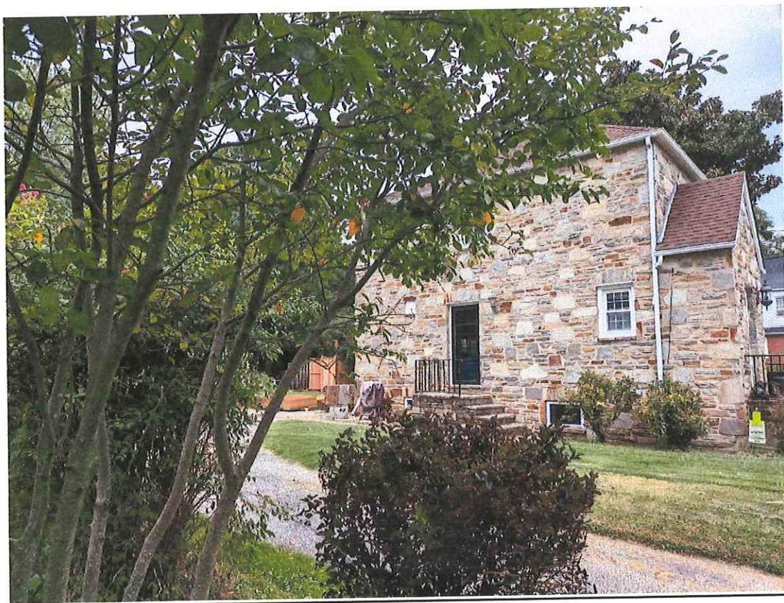
Adjacent property at 2022 Rocky Point Road
