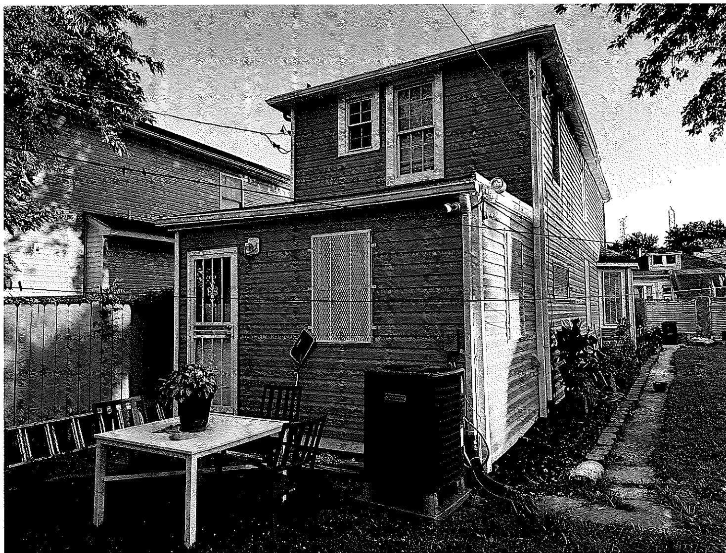
Rear of the house
