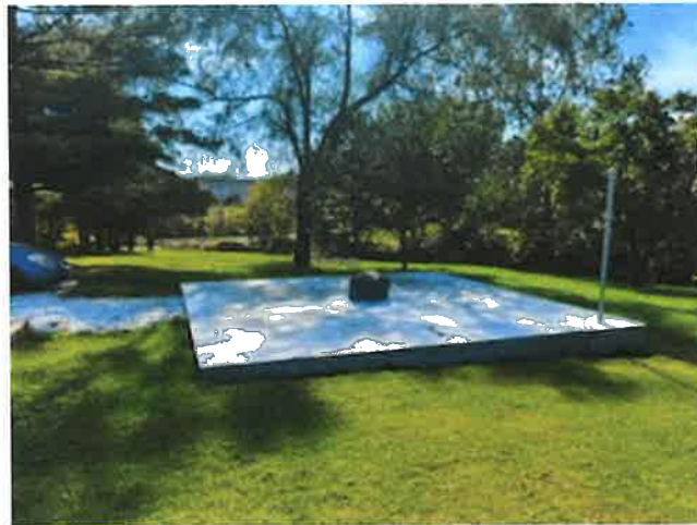
Side view From Carport
