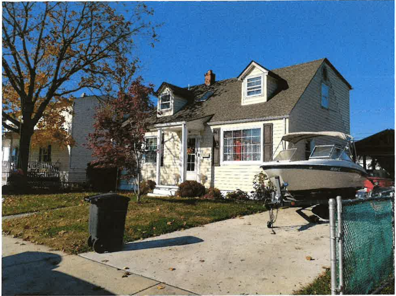
PHOTOGRAFY RIGHT SIDE
