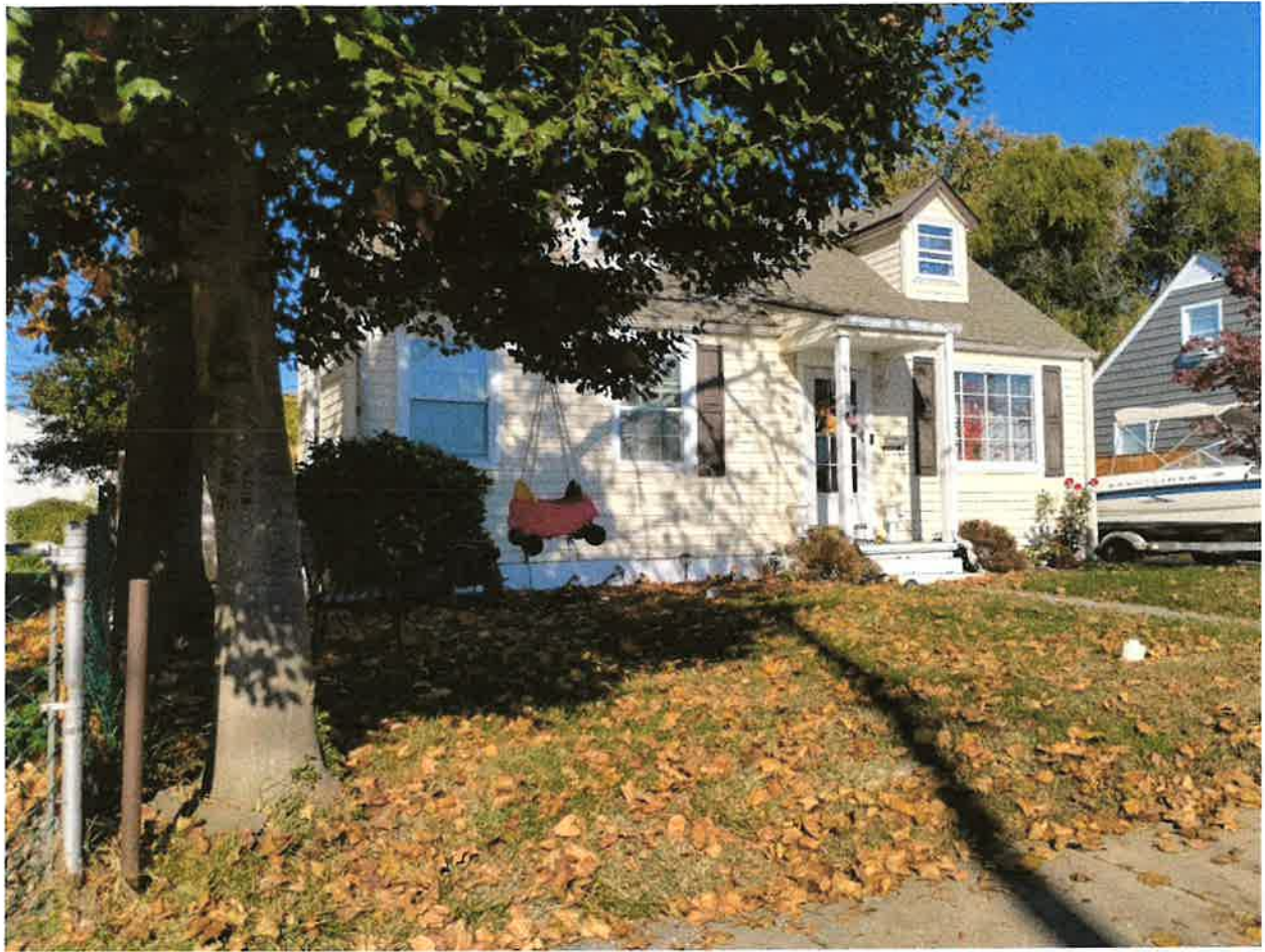
PHOTOGRAFY LEFT SIDE OF THE HOUSE
