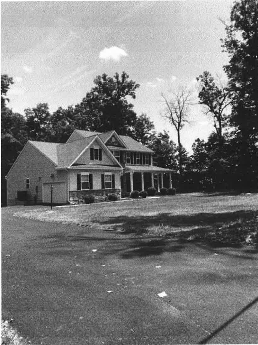
FRONT VIEW PROPERTY
