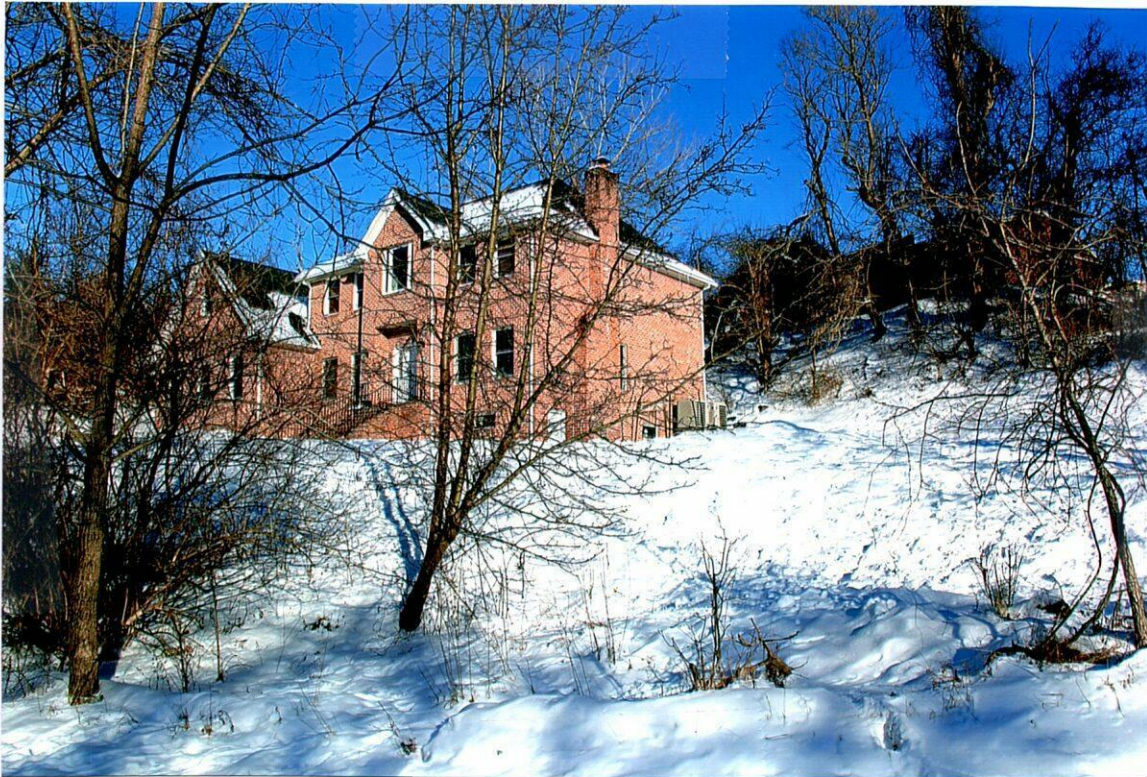
RIGHT SIDE VIEW ILLUSTRATING THE STEEPNESS OF THE LOT AND HILL IN REAR
