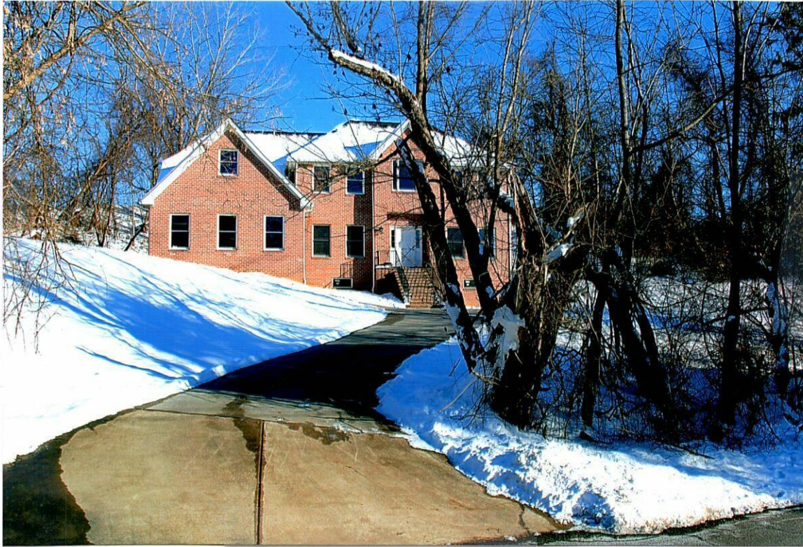
FRONT VIEW ILLUSTRATING THE STEEPNESS OF THE LOT AND DISTANCE FROM THE ROAD
