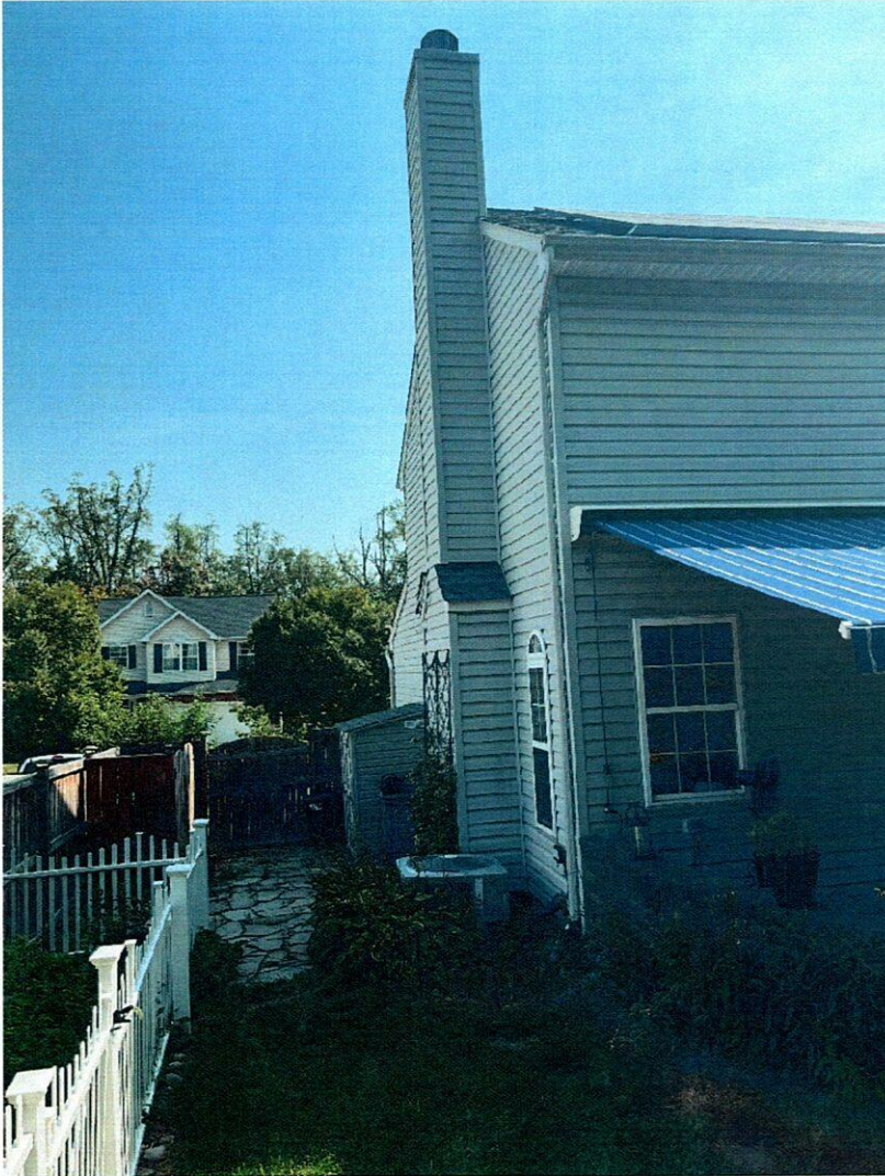
North side of house, looking toward Oakdale Ave
