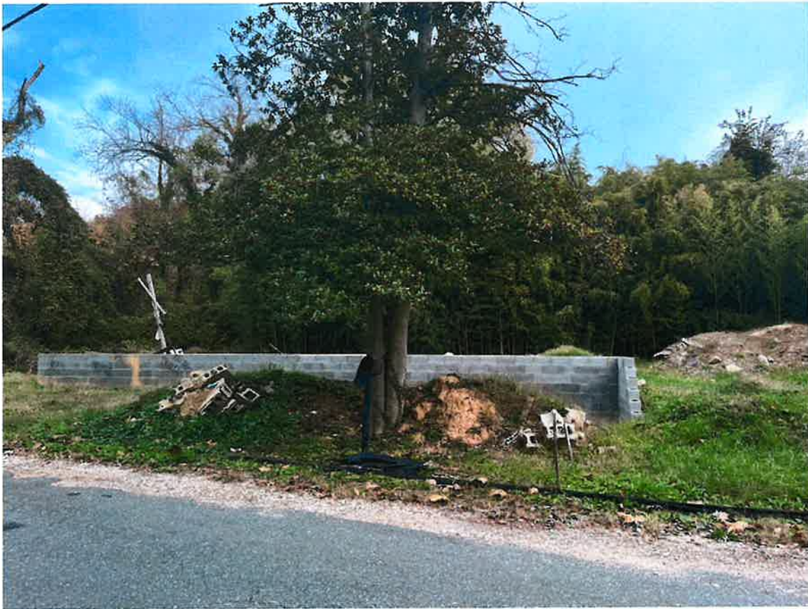
Photo 3: Existing/current structure building – Front Side along Jeanne Ave
