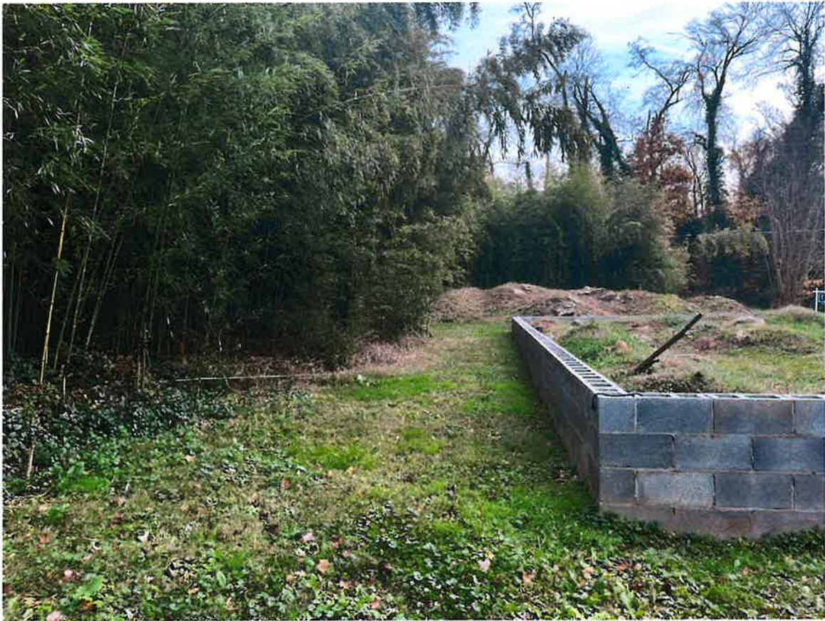
Photo 5: Existing/current structure – back yard (eastside) from Jeanne Ave
