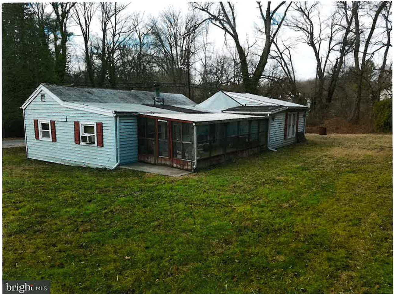
Photo 2: Existing demolished building – Back Side
