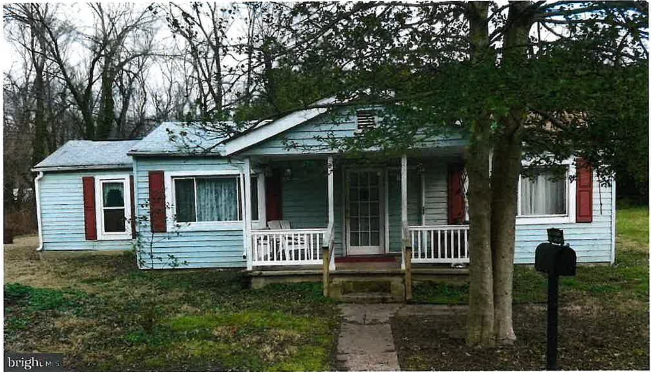
Photo 1: Existing demolished building – Front Side
