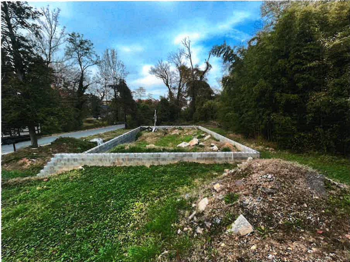
Photo 6: Existing/current structure – From Arline Ave.
