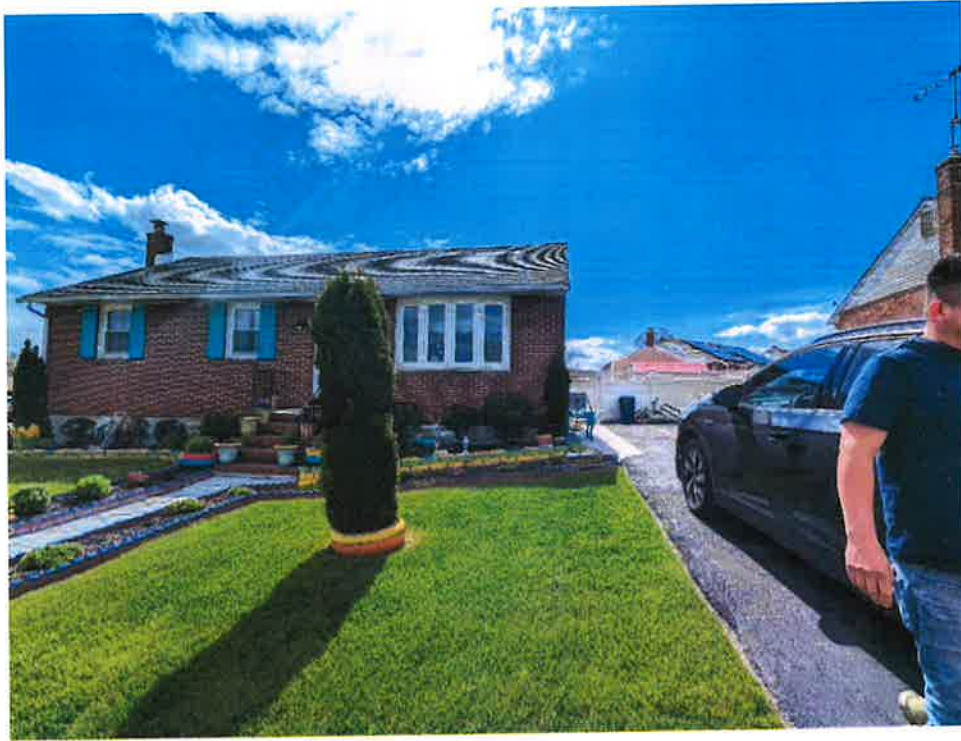
Street view of 1502 Chesaco Ave. Proposed carport to be on right side of existing SFD.
