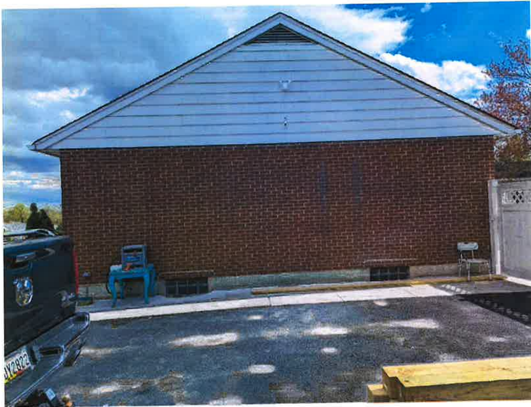
Right side of existing driveway and SFD.
