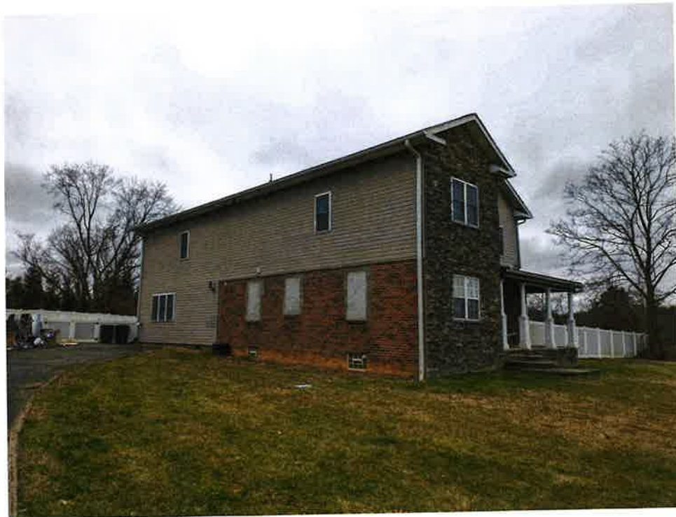
Side view of existing residence
