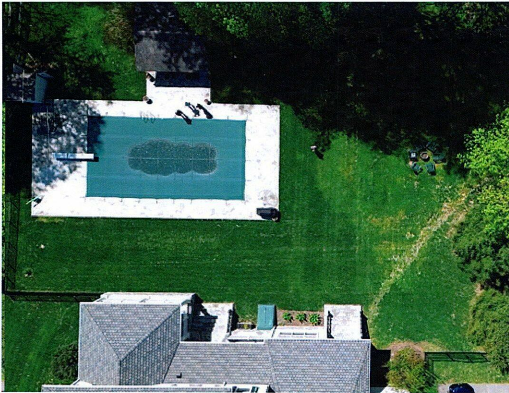
Aerial view of the existing pool, pool house and back ½ of the main house
