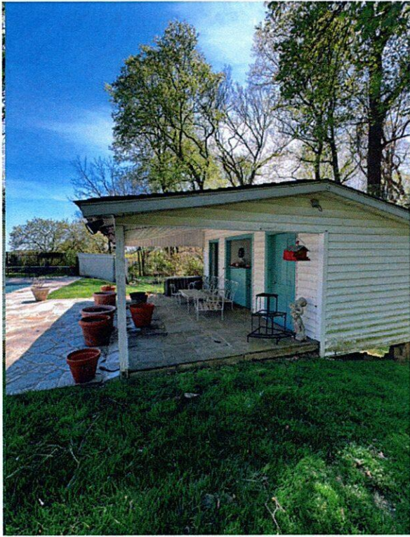
Right side of the existing pool house
