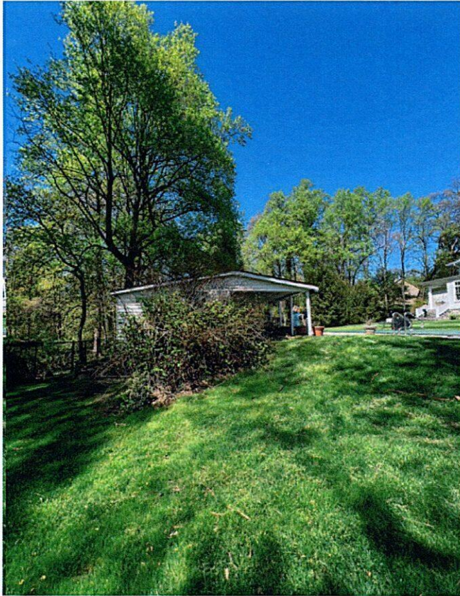
Left side view of the existing Pool house
