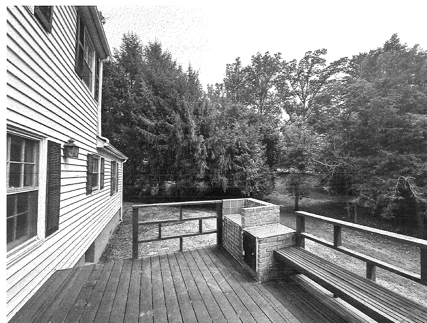
VIEW FROM EAST LOOKING NORTH
