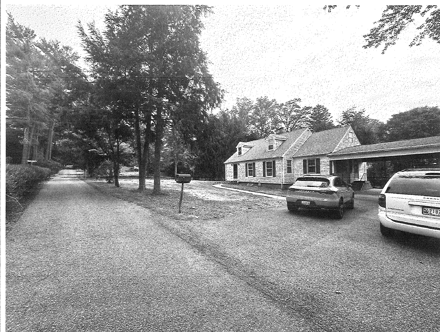
APPROACH FROM SOUTH WEST
