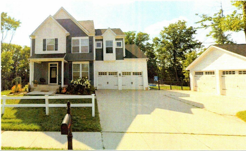
Front view of existing residence
