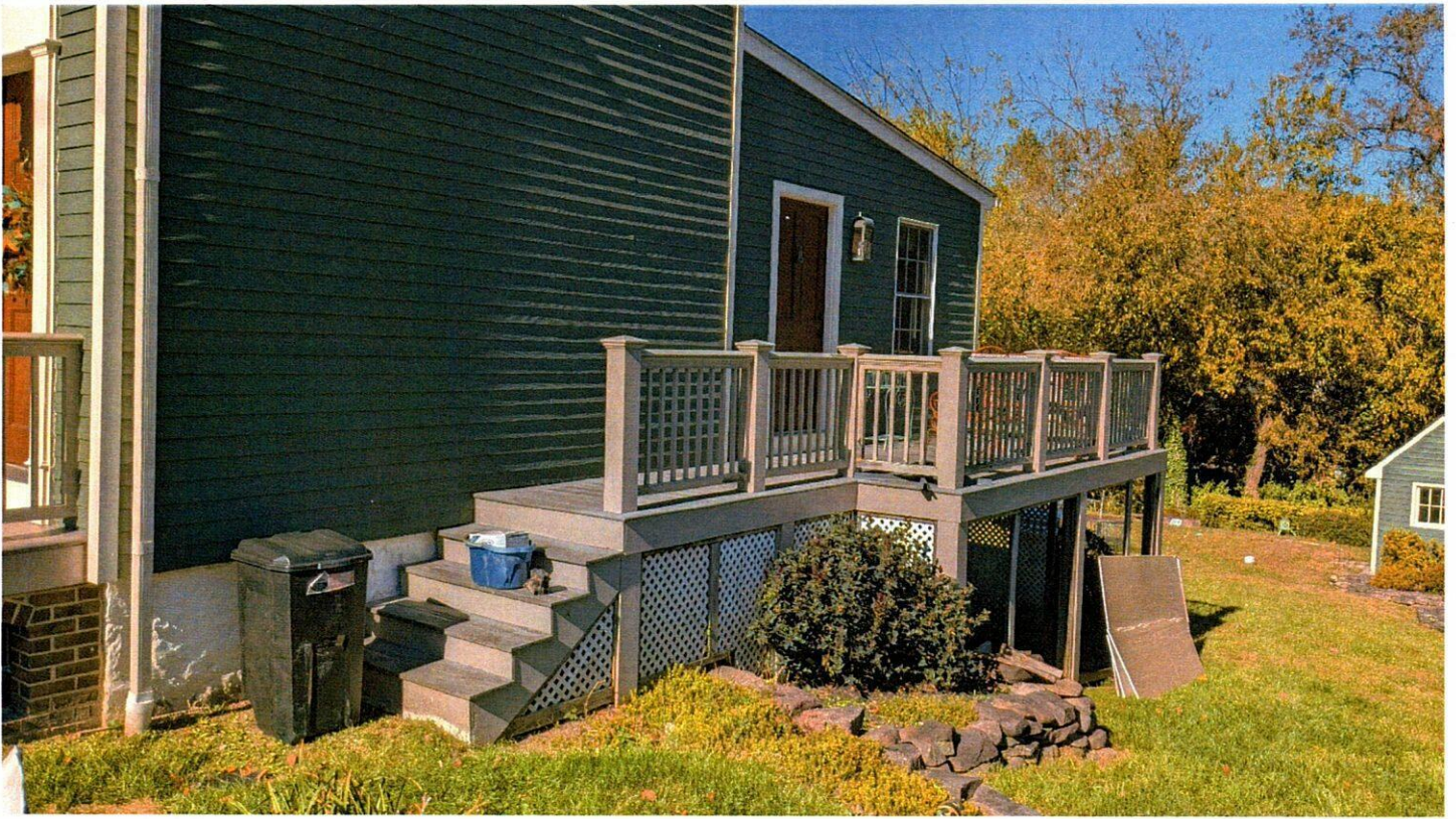
Existing Right Side Deck View
