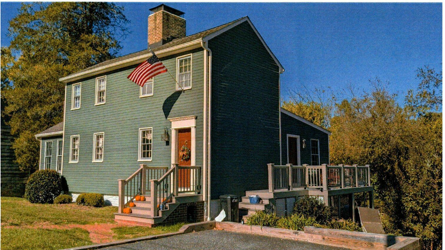
Street Front Right Side View
