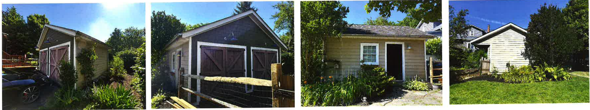
REFERENCE PHOTOS OF EXISTING STRUCTURE TO BE RENOVATED
