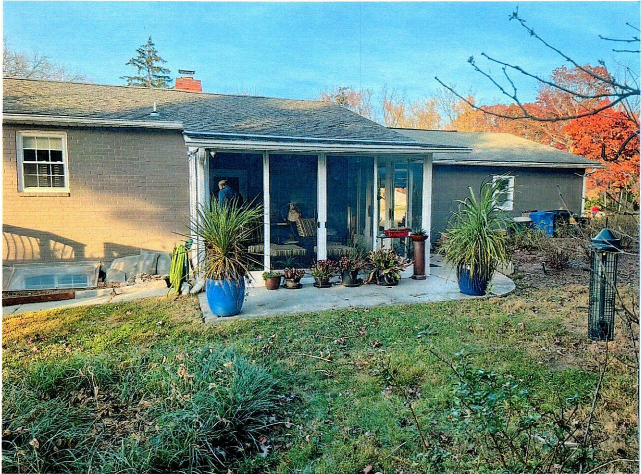
View of existing sunroom where the larger sunroom will be located
