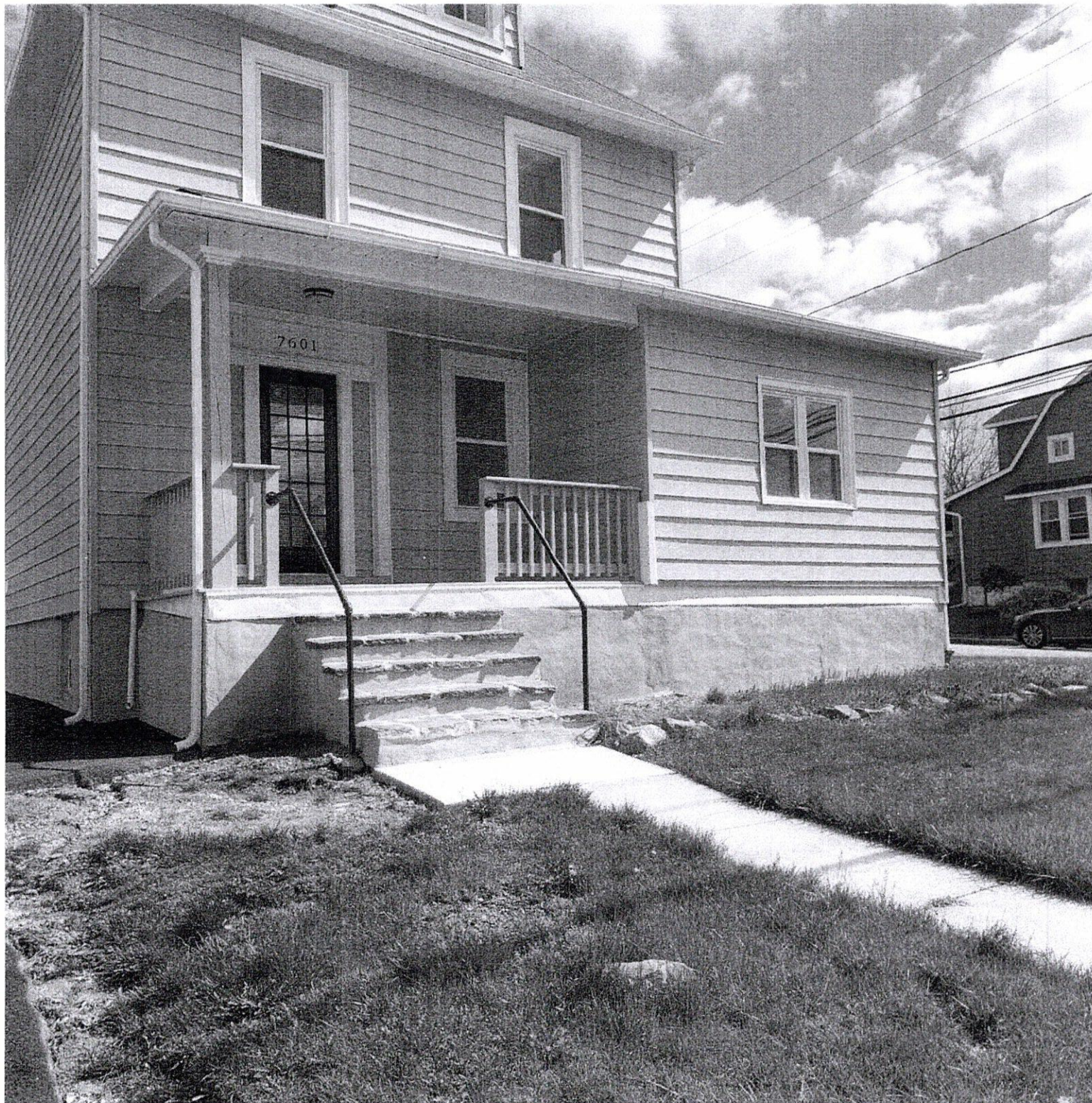
FRONT VIEW FROM OLD HARFORD ROAD
