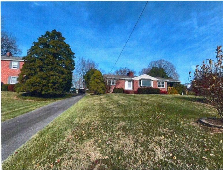
Front of house, neighbor on left (west)
