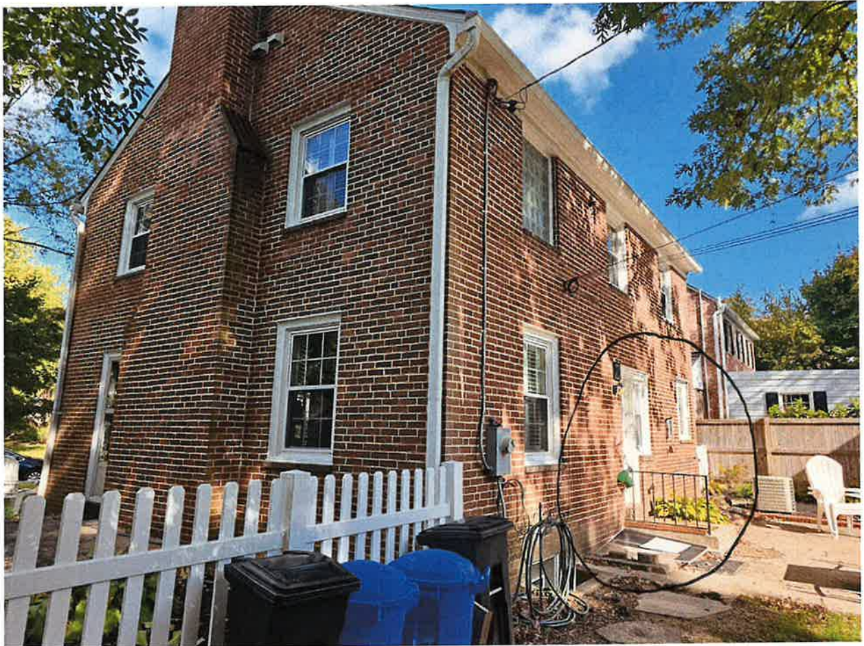
Orr Basement and Kitchen Egress
