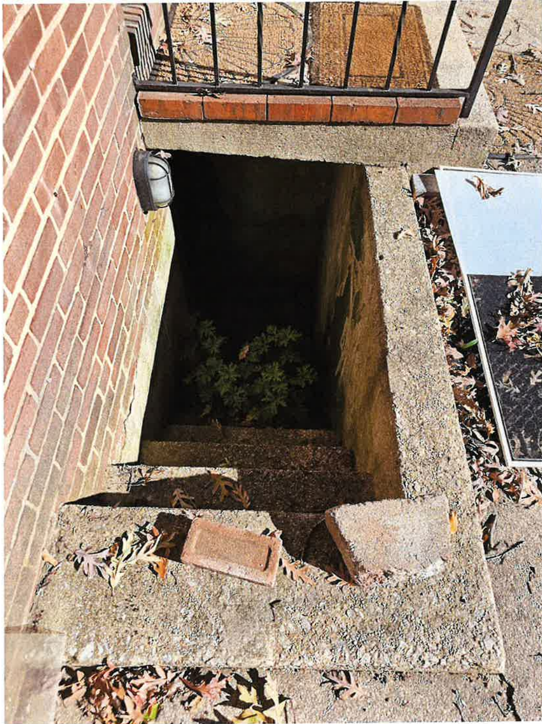
Close up of Basement Egress with Kitchen Door Egress above
