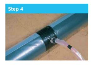
Wrap any connected copper service line within three (3) feet of the pipe with polyethylene or dielectric tape.
