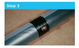
After making the direct service connection, inspect the entire circumferential area for damage and make any necessary repairs.
