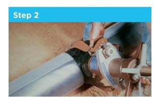
Mount the tapping machine on the pipe area covered by the polyethylene adhesive tape. Then make the tap and install the corporation stop directly through the tape and polyethylene.
