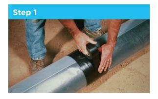
Wrap two or three layers of polyethylene adhesive tape completely around the pipe to cover the area where the tapping machine and padded chain will be mounted.
