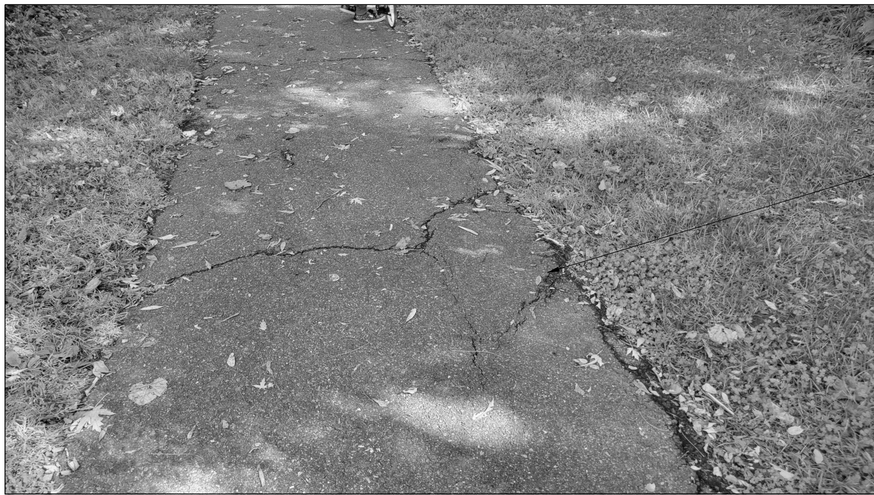
REPAIR TYPE 2 : SEAL LINEAR CRACK REPAIR
