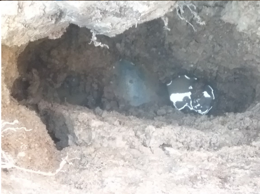
Test Pit TP-1 Existing 8" Steel Water pipe
